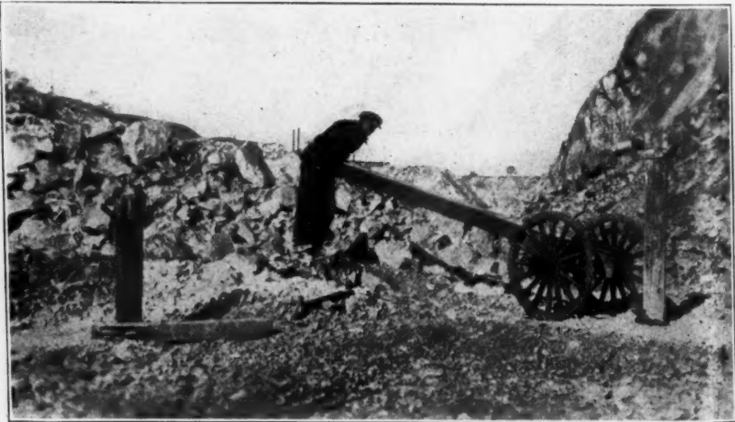
Device for Pulling Up Blast Hole Casings
